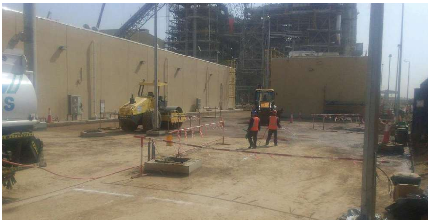
Control Building Site Preparation, Jazan IGCC
