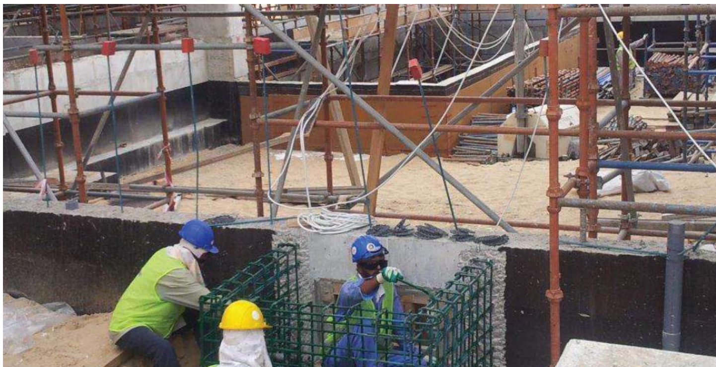
Data Centre Building, Sadara Jubail
