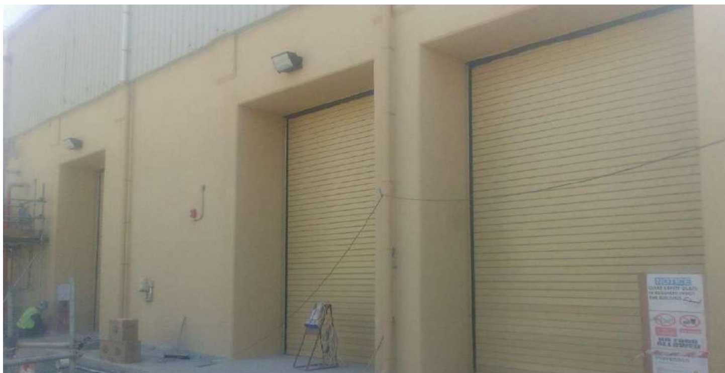
Warehouse & Workshop Building, Jazan IGCC
