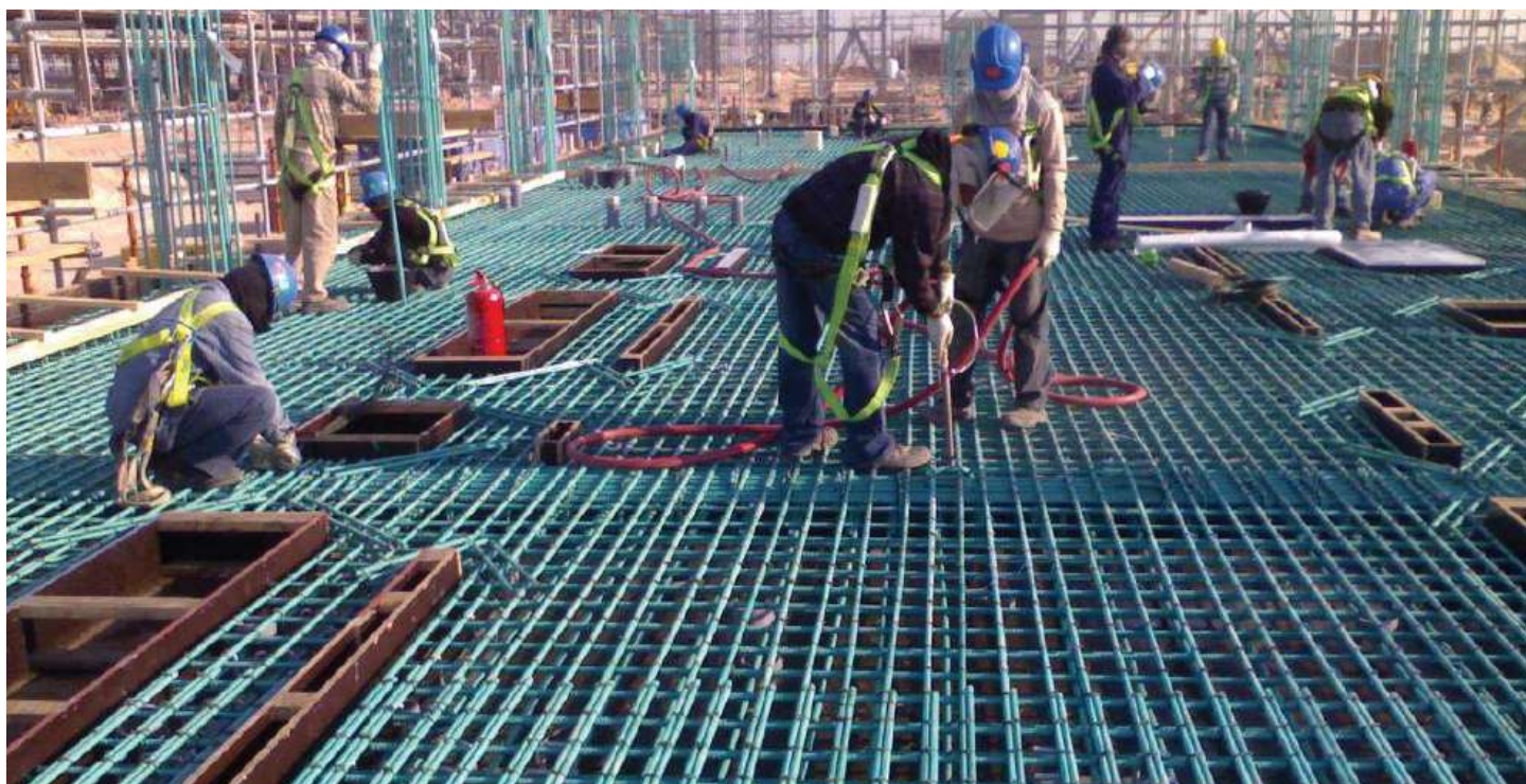
Data Centre Building, Sadara Jubail
