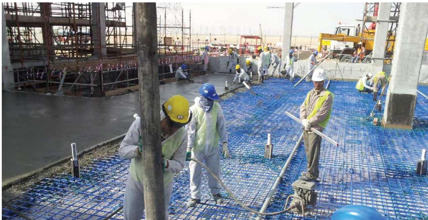
Data Centre Building, Sadara Jubail
