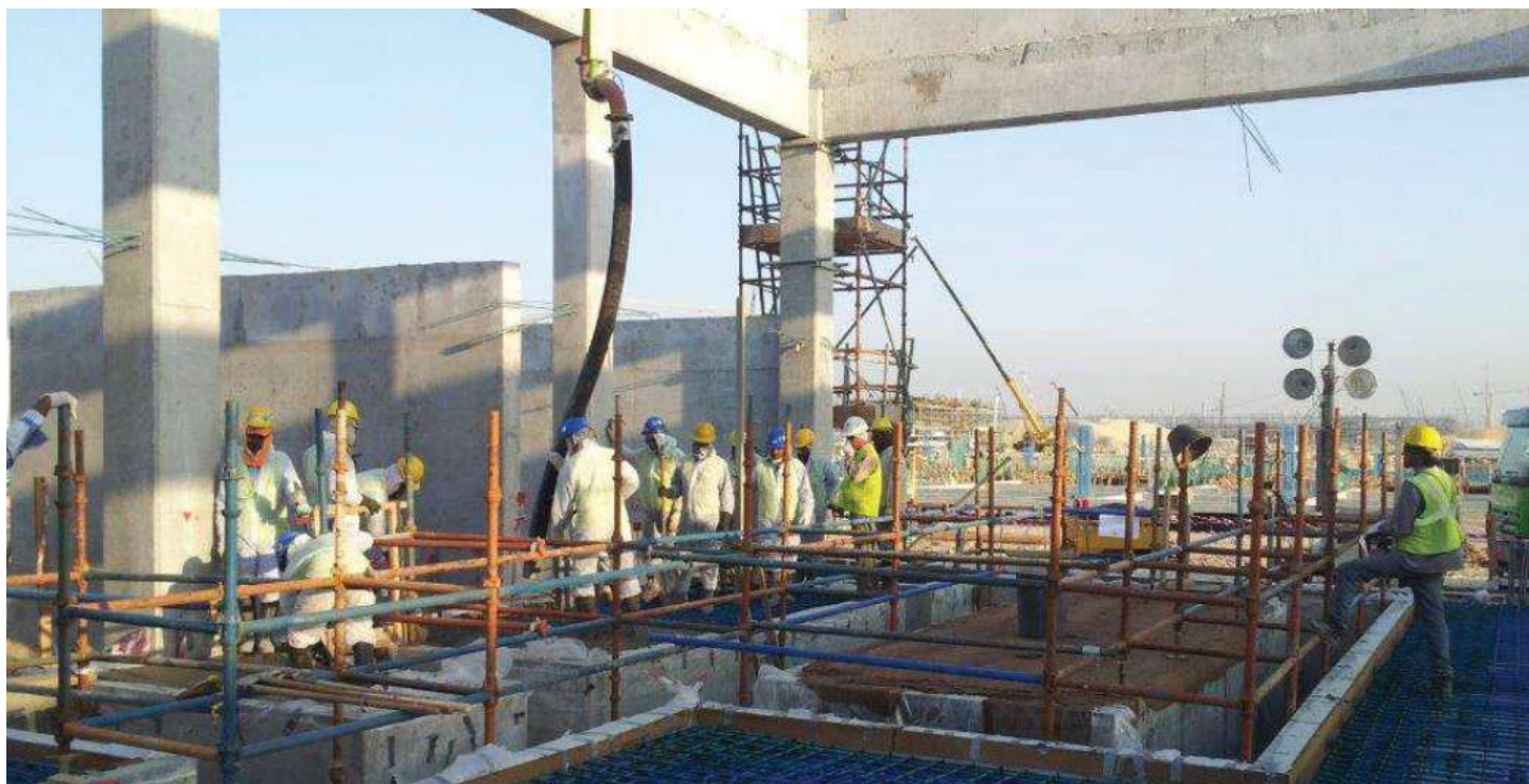
Data Centre Building, Sadara Jubail
