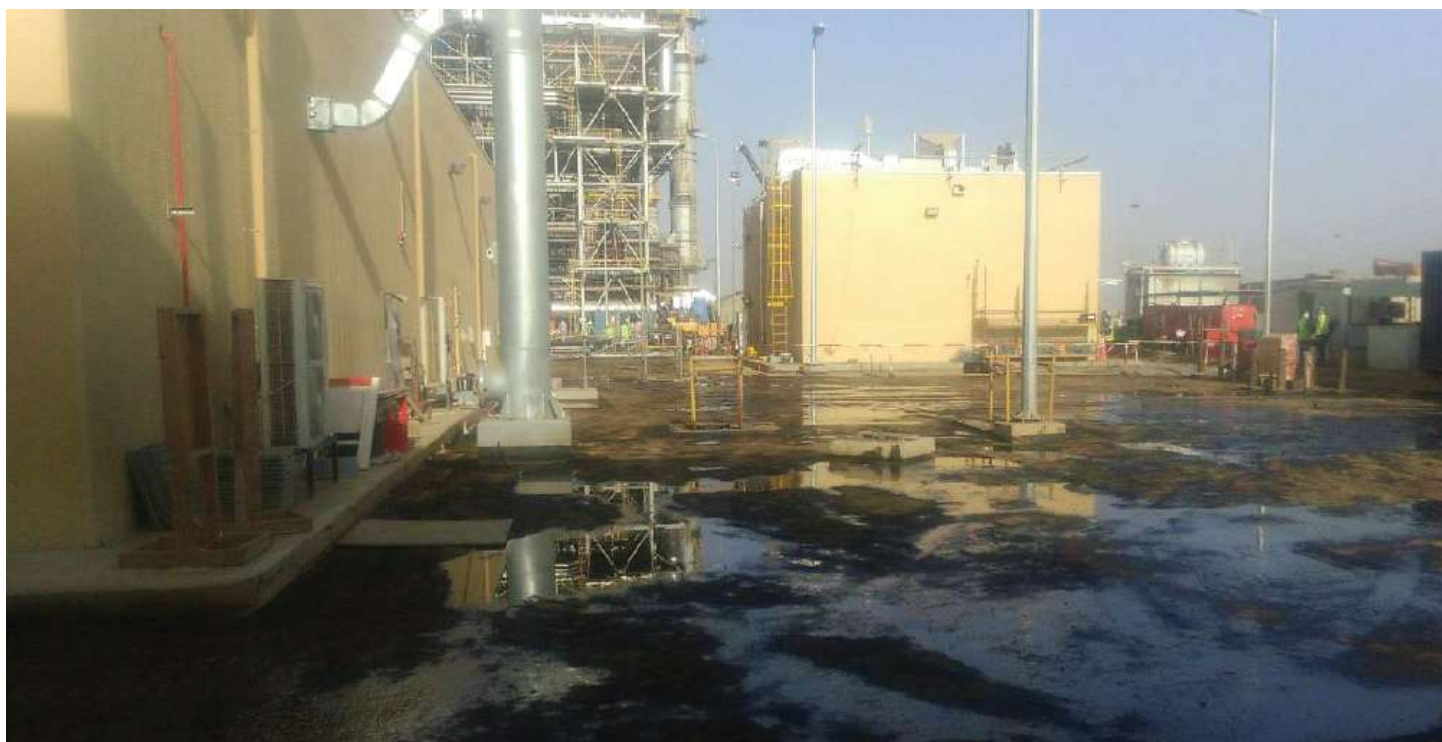
Control Building Road Paving, Jazan IGCC
