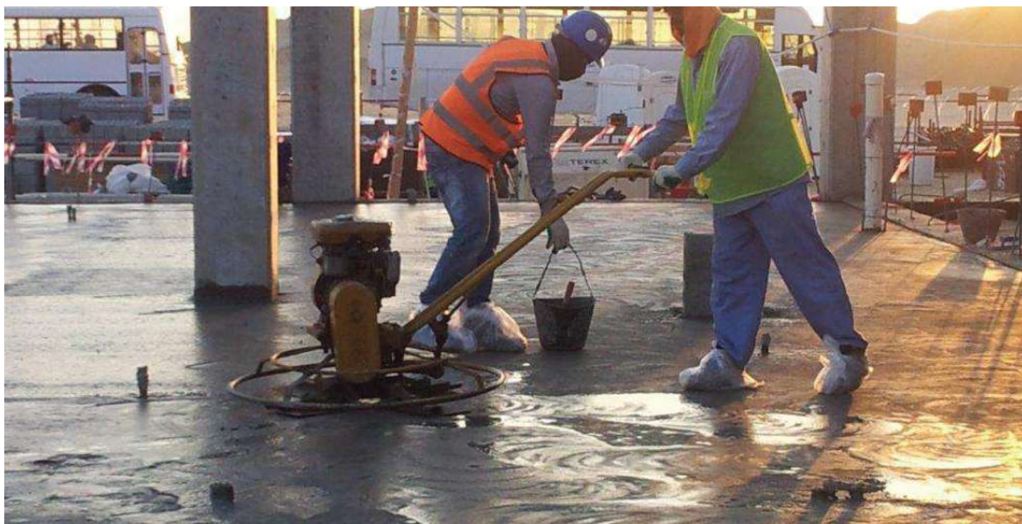
Data Centre Building, Sadara Jubail
