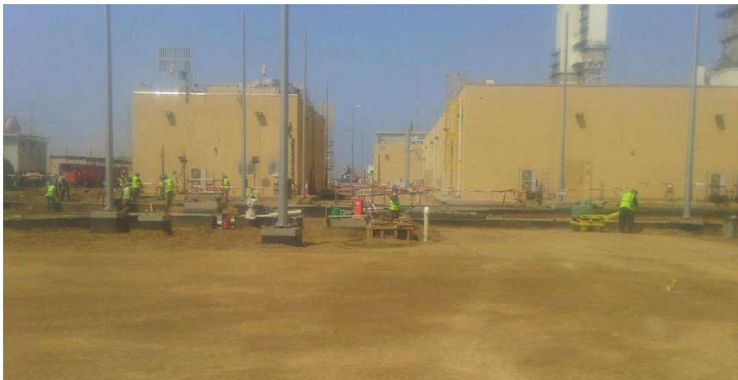
Security & Guard House Building
