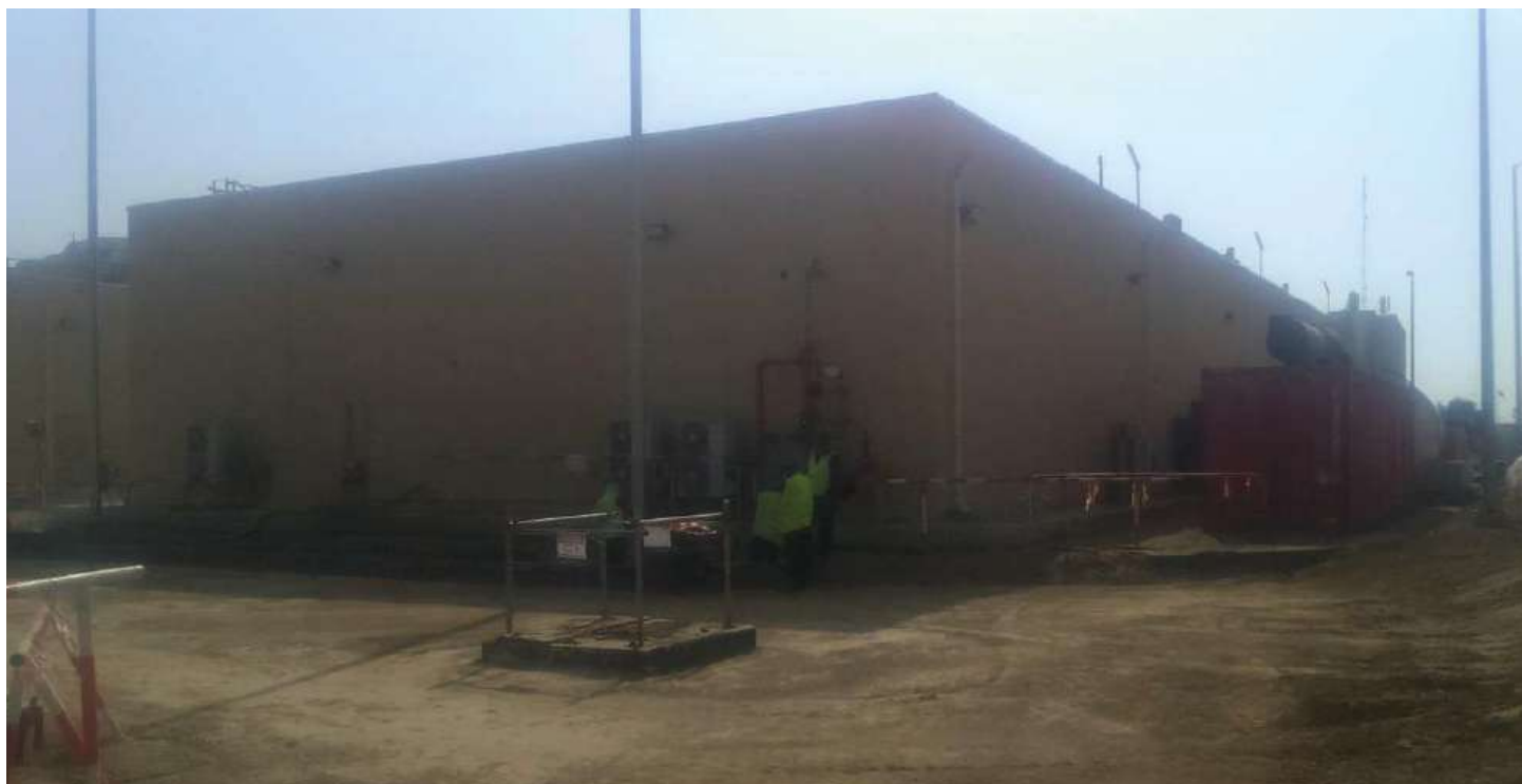
Control Building Site Preparation, Jazan IGCC
