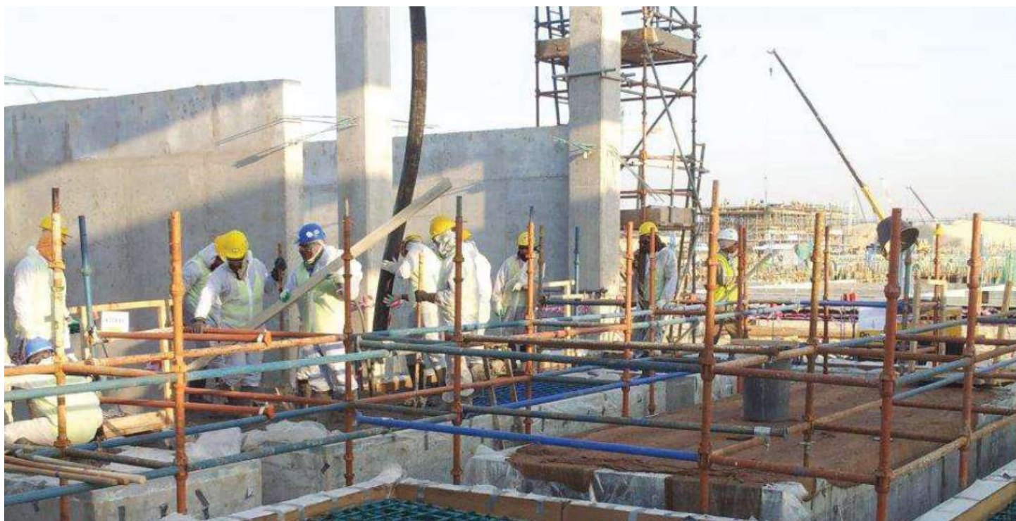
Data Centre Building, Sadara Jubail
