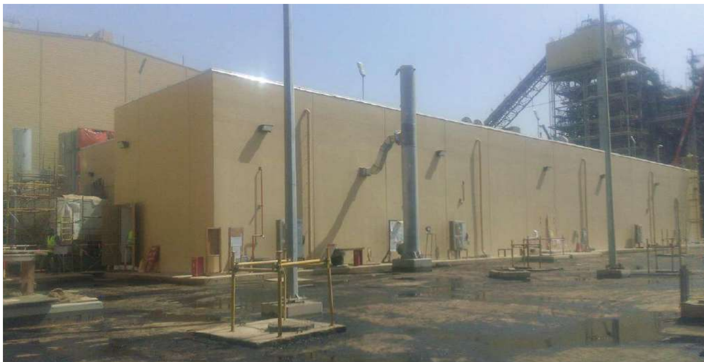
Control & Admin. Building, Jazan IGCC
