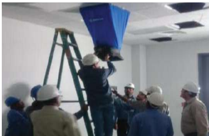
Testing and Air Balancing
